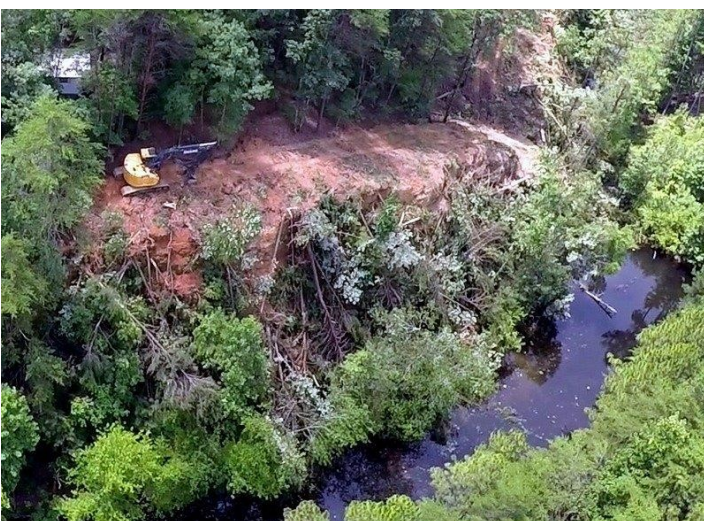
Three Forks, South AML Reclamation Project in Tuscaloosa County at the start of construction.
